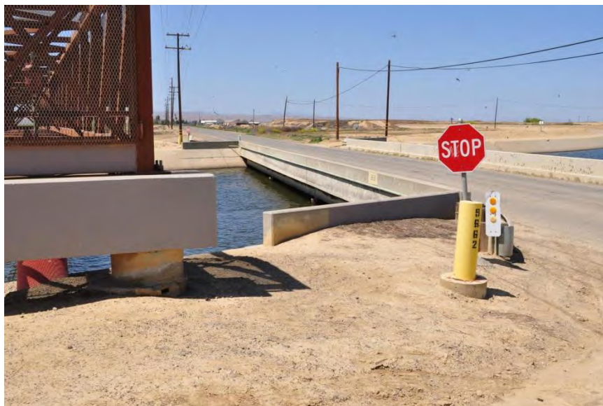
Figure 4-16. Delta Mendota Canal at Athena Road north from Mendota, CA; downstream is to the left. The bridge has experienced a substantial loss of clearance as the land subsided.
