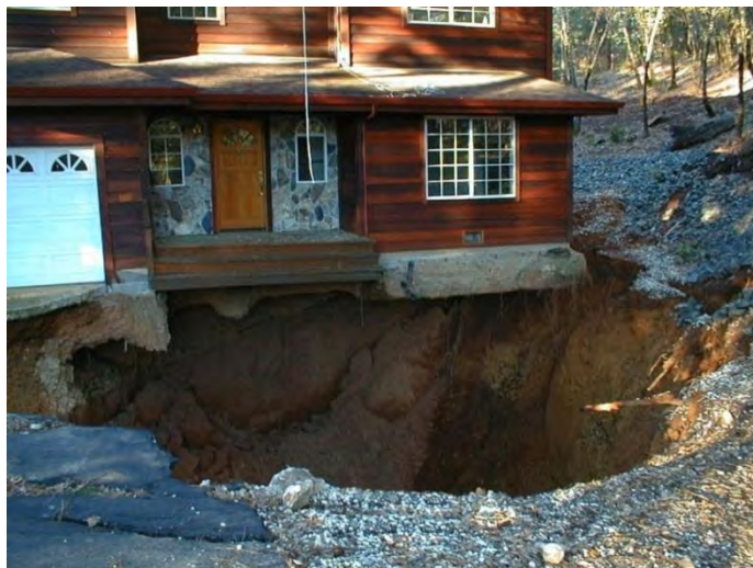
Figure A-1. Collapse into the Old Brunswick Mine, Grass Valley, California (photo courtesy of California Department of Conservation).
