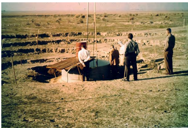
Figure A-6. Concentric tension fissures and differential subsidence resulting from hydrocompaction at a 6-ft diameter corrugated infiltration test pit on the proposed alignment of the California Aqueduct, December 12, 1960.
