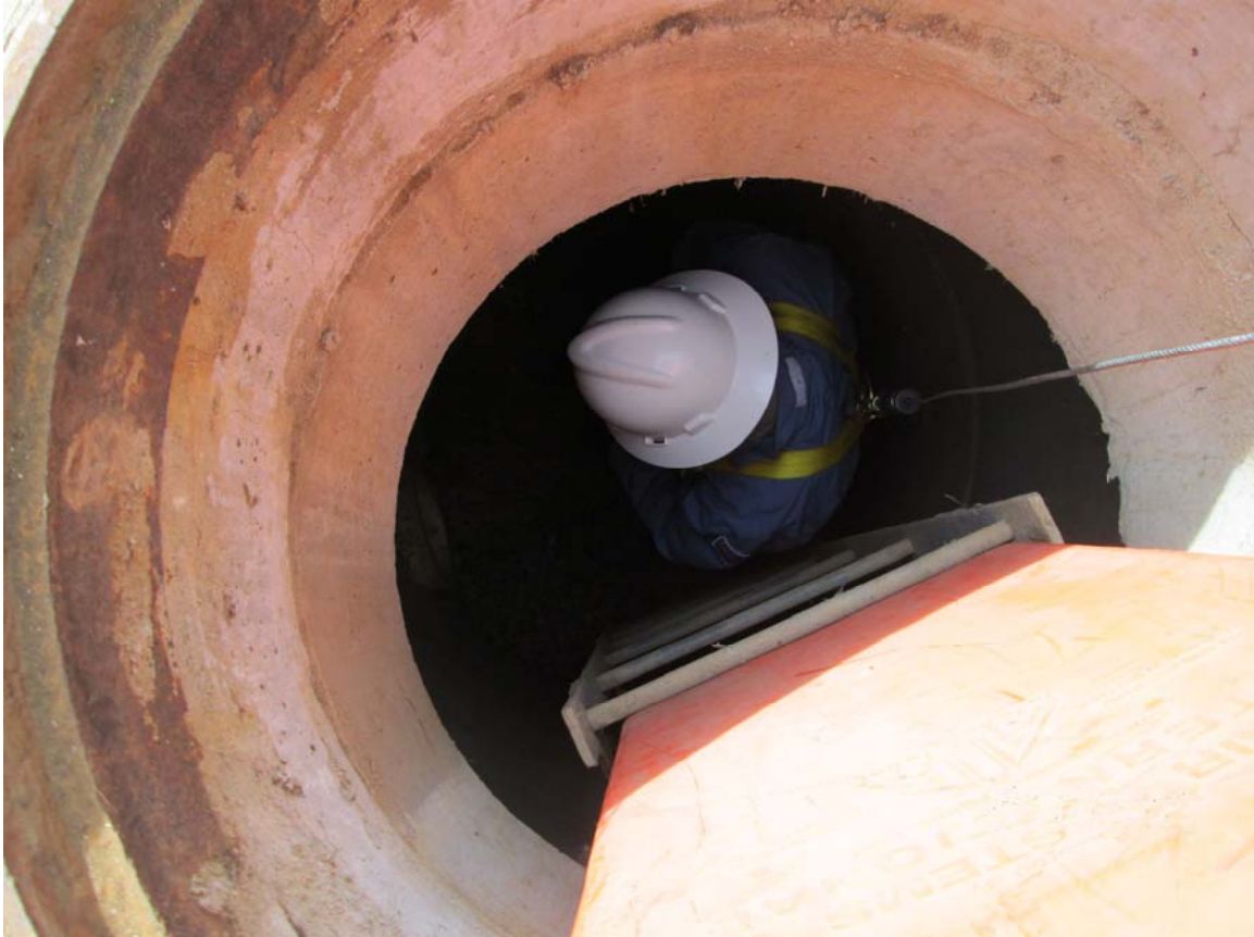
Staff accessing vault for inspection 2019
