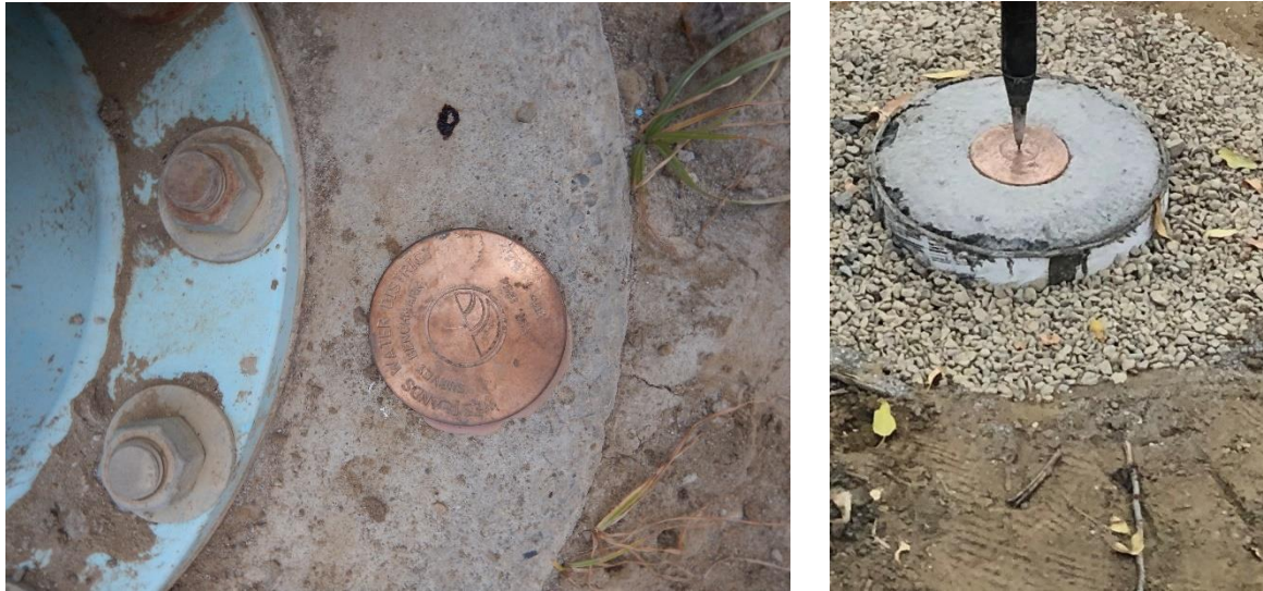
Figure 1. Monument set in Meter Base (left) and Monument set in 10" concrete(right)
