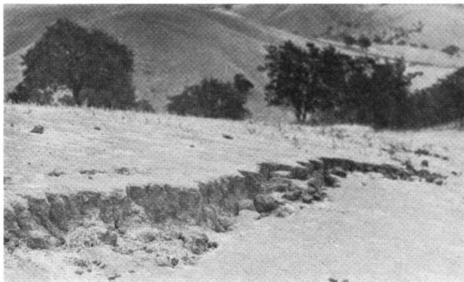
Photo No. 15—Offset of ground surface north of U. S. Highway 466 near the Bealville turnoff. Offset is one foot with the northwest side up. Much of this movement is probably due to slump.
