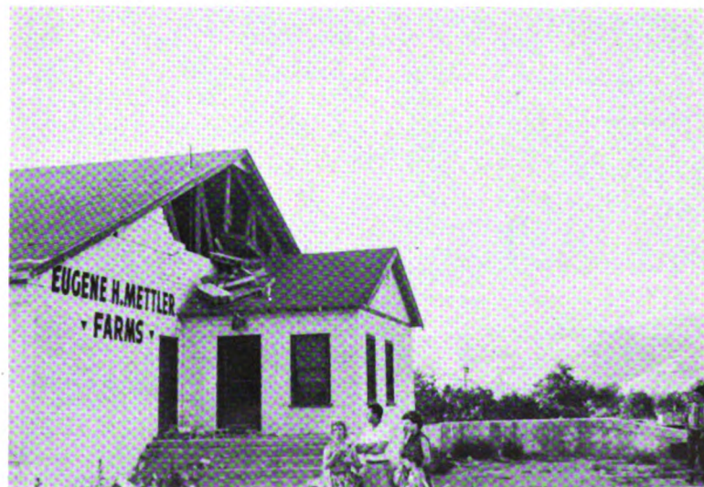
Photo No. 31—Brick building across street from previous photo showing good brick construction with bond beams. A few bricks fell as a result of racking of wooden truss roof. Photo by Division of Architecture.
