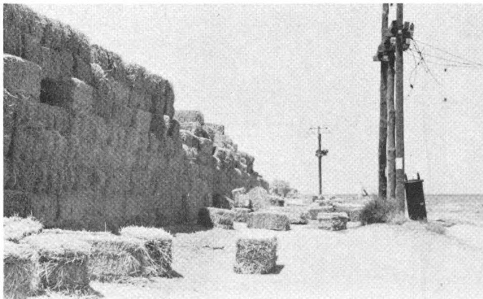
Photo No. 4—Haystacks and transformers toppled about 15 miles south of Bakersfield along U. S. Highway 99.
