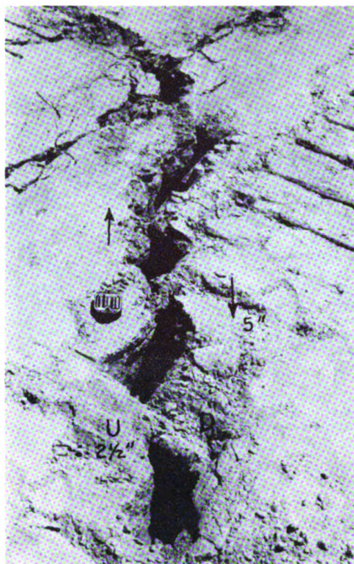
Photo No. 1—A northeast trending crack in a dirt road about 15 miles south of Bakersfield. Movement is as noted. View is looking northeast.
