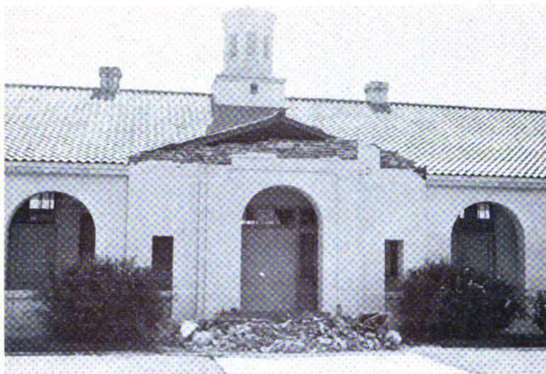
Photo No. 11—This school located about five miles west of Arvin was in the megaseismic area. Two stone ornaments insecurely fastened on either side of archway rocked loose and pulled out a few bricks. Balance of school undamaged.
