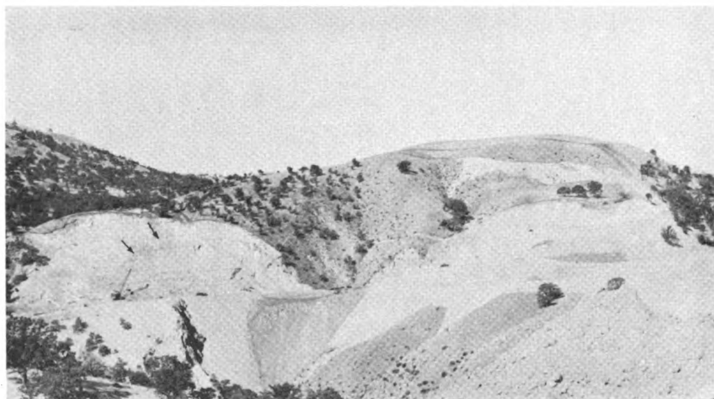
Photo No. 16—View looking southwest toward former location of Southern Pacific Tunnel 4 on left and Tunnel 3 on right located south of Caliente. Note dark zone dipping 43 degrees to east in cut above Tunnel 4. This zone is a fault breccia with gouge matrix. Some movement probably took place along this zone for Tunnel 4 was damaged severely where this zone intersected the bore.
