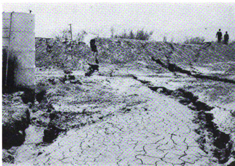
Photo No. 2—Northwest trending cracks near a reservoir about 15 miles south of Bakersfield. Cracks have been widened by water pouring from the reservoir.
