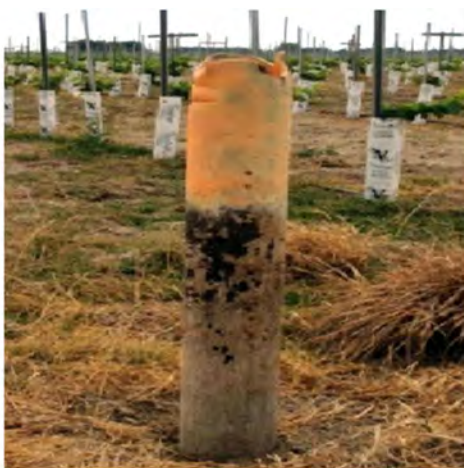
Figure 4-22. Well casings protruding from land surface just south from El Nido. Left: casing of an abandoned gas well protrudes more than 46 cm (1.5 ft) higher than when it was painted 2 years earlier. Right: protruding casing of an irrigation well lifts its concrete surface pad and piping off the ground as land settles around it (photographs courtesy of Chris White, Central California Irrigation District).
