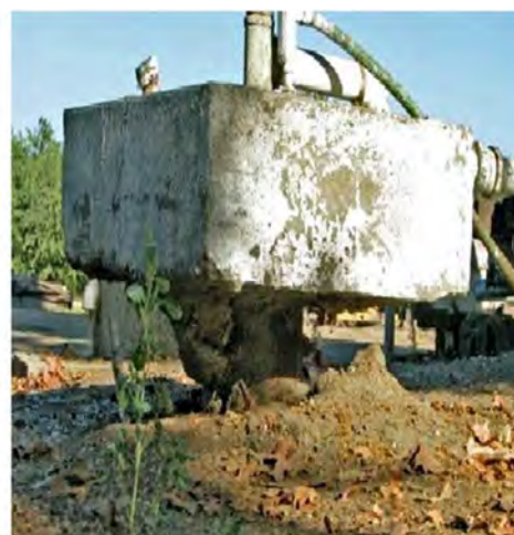
Figure 4-22. Well casings protruding from land surface just south from El Nido. Left: casing of an abandoned gas well protrudes more than 46 cm (1.5 ft) higher than when it was painted 2 years earlier. Right: protruding casing of an irrigation well lifts its concrete surface pad and piping off the ground as land settles around it (photographs courtesy of Chris White, Central California Irrigation District).
