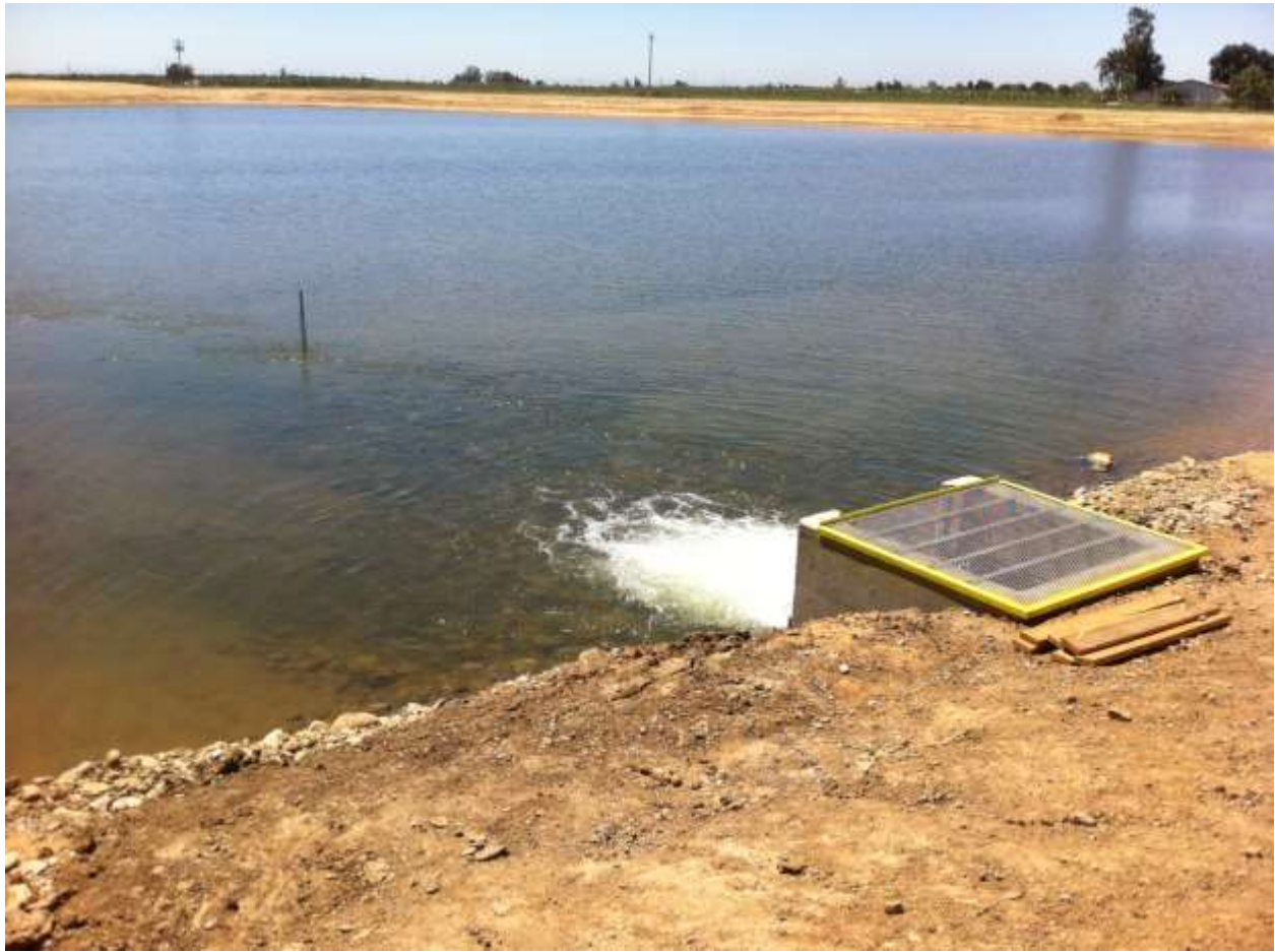
CRESSEY RECHARGE BASIN
