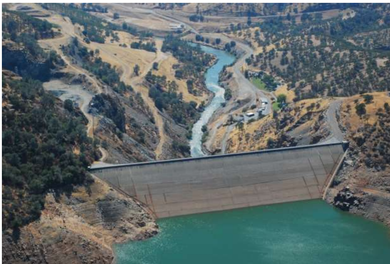
NEW EXCCEQUER DAM
