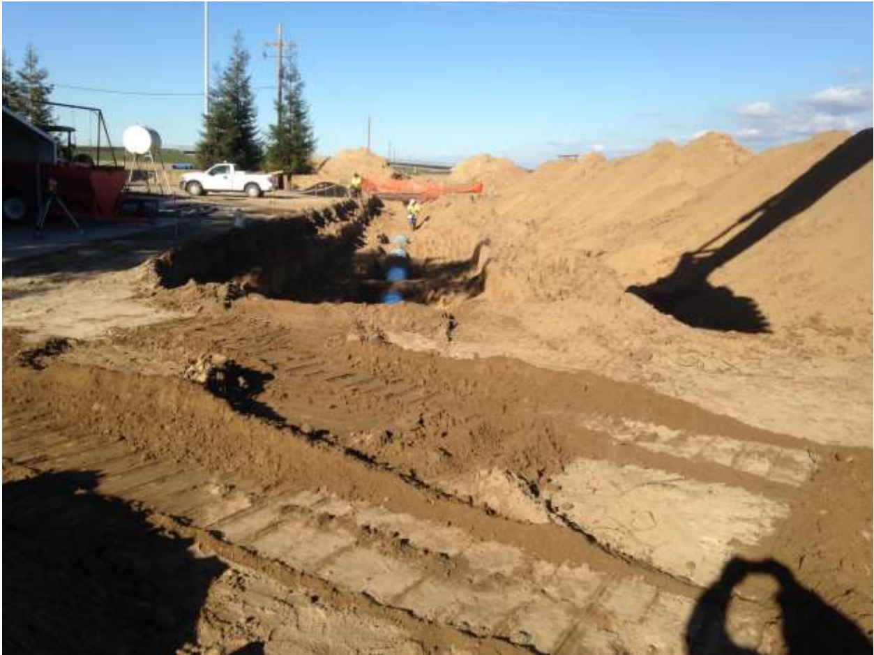
HIGHLANDS 10,000 LF PIPELINE INSTALLATION
