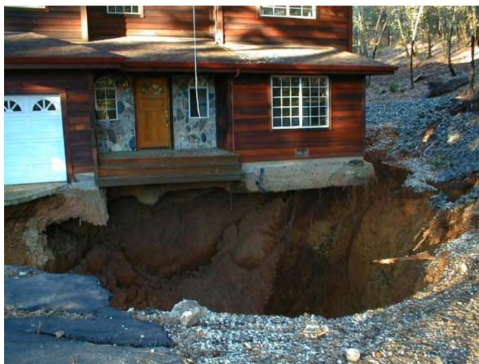
Figure A-1. Collapse into the Old Brunswick Mine, Grass Valley, California (photo courtesy of California Department of Conservation).
