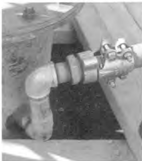
Figure 15.24. In the pressurization method, the eductor and air line are placed in the well and then the casing is capped. (Bergerson-Caswell, Inc.)
