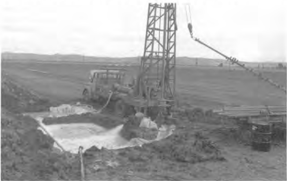
Figure 10.12. Drilling fluid from the borehole flows into the larger pit where the cuttings settle out. The fluid then flows into the second pit through a constricted opening. The mud pump on the rig withdraws drilling fluid from this pit to inject down the drill rods to the bit. This Italian driller has lined the drilling fluid pits with polyethylene film to reduce fluid loss into the ground. Note the homemade hole cleaner or scratcher the driller uses to keep the borehole open during drilling.
