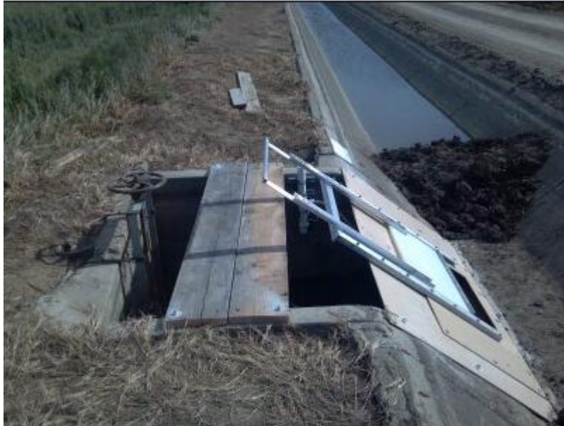
Figure 7.2: Fixed Orifice Plate
