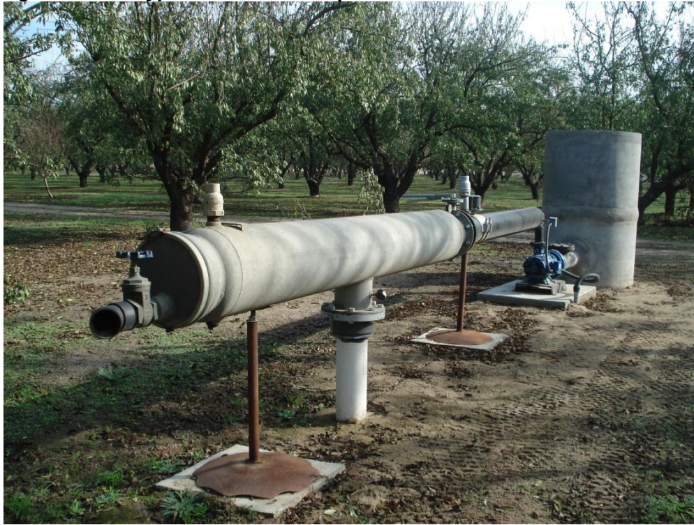
Figure F-4 Typical Booster Pump Installation
