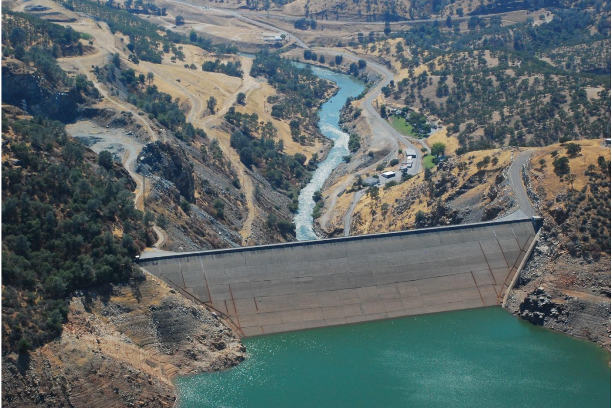
New Exchequer Dam
