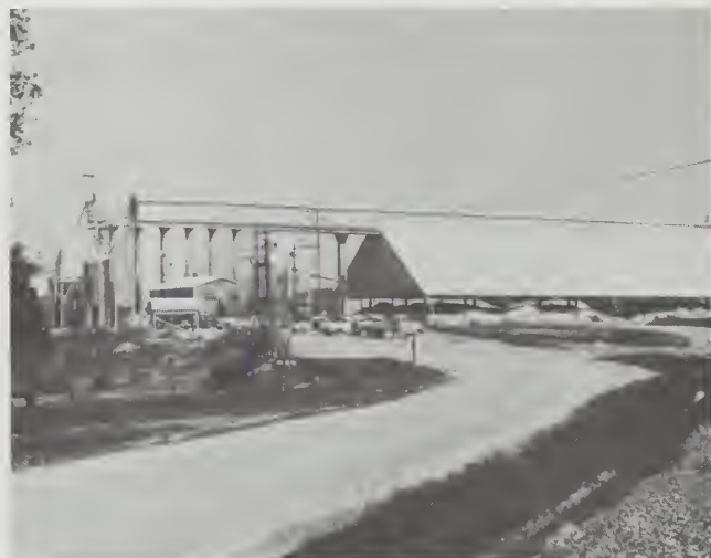
Photo 7. Interpace Corporation Indian Hill clay plant, located about 3 1/2 miles northwest of Ione.
