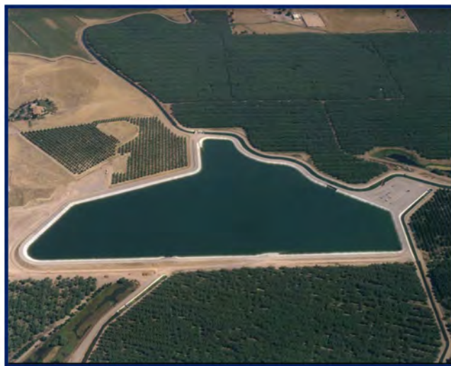
Figure 3-4. North Side Regulating Reservoir.
