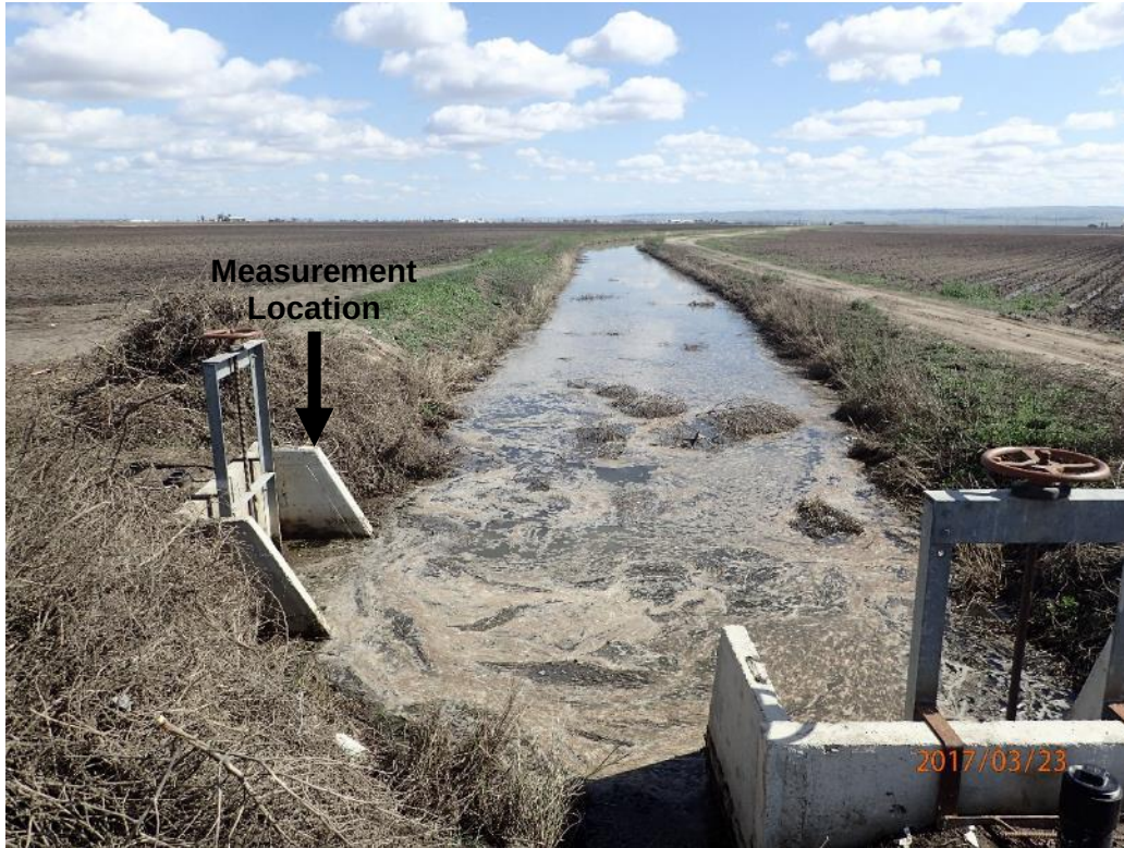
Figure 6 – Angelo Canal looking southeast from northern end. Note two canal gates, both with slow leaks, and measurement location.
