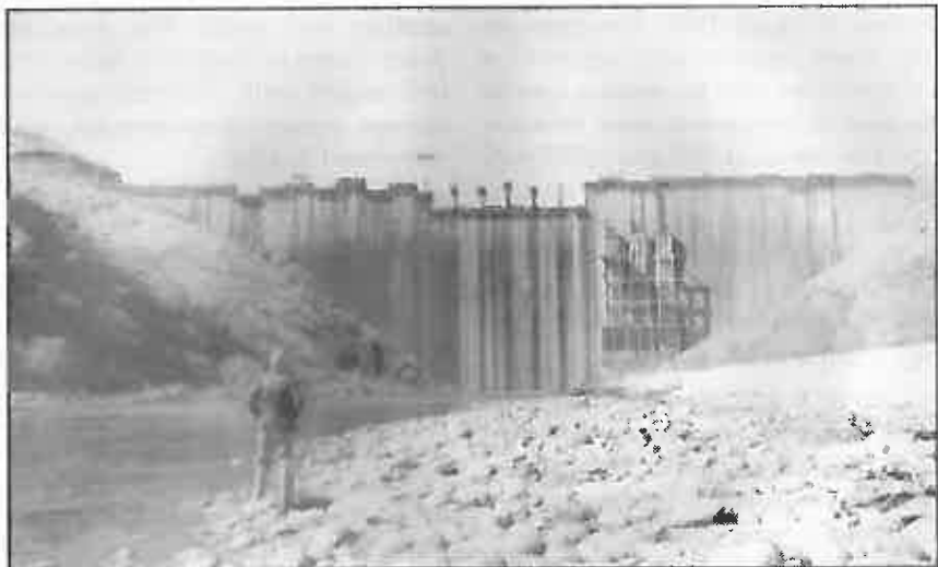
This upstream picture of Pine Flat Dam during construction shows the penstock intake structure on the right that were built for the future construction of a power plant.
