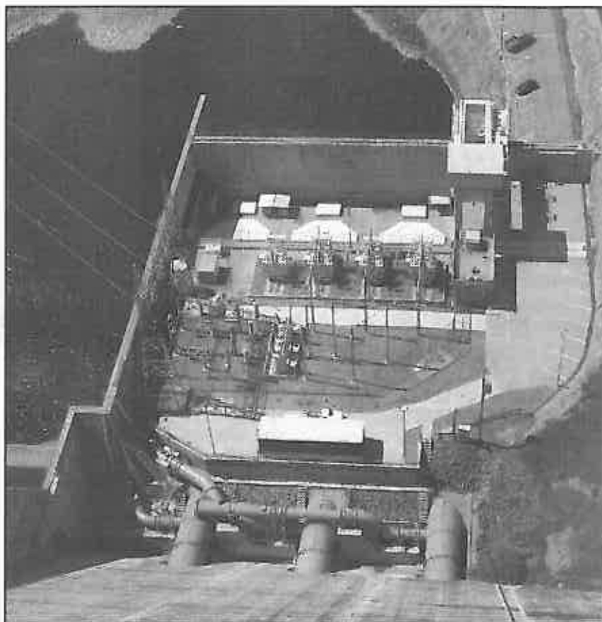
Looking down from the top of the dam at the Jeff L. Taylor-Pine Flat Power Plant. The large pipes emerging from the dam are penstocks carrying water to the turbines. The smaller pipe system at the dam's base is part of the new turbine bypass.
