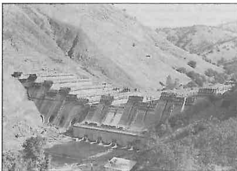
Pine Flat Dam takes shape in 1950. The concrete gravity dam was built in blocks 50 feet wide and five feet high.
