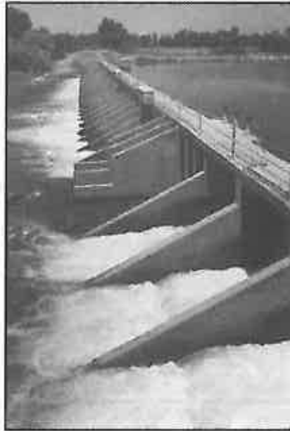
Peoples Weir, located a mile downstream from State Route 99, is the largest such structure on the Kings River. Water is diverted here into portions of Kings County.
