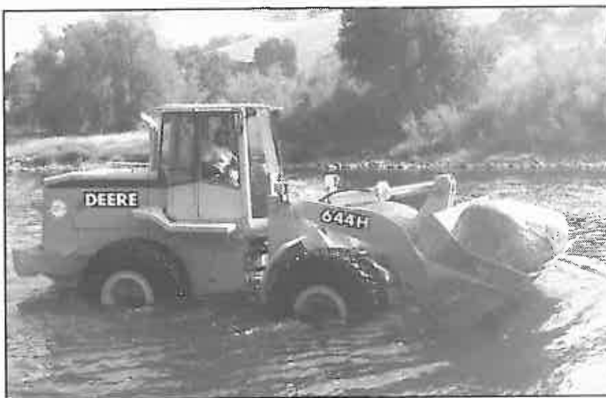
Boulders by the thousands have been placed in the channel for enhanced habitat under the Kings River Fisheries Management Program.
