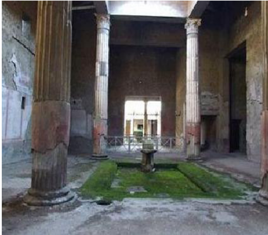
Figure 2 Ancient Rainwater Harvesting Techniques in Pompeii Consisted of an Impluvium Designed to Direct Rainwater to an Underground Cistern (Photo Credit: Jan Walker)
