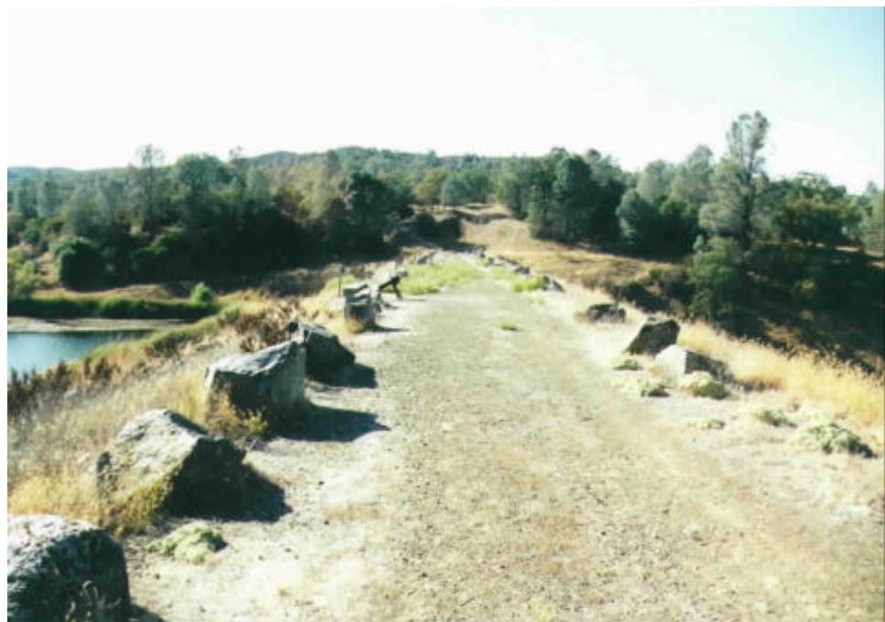
Photograph 6-5 Highland Creek Dam looking west along the crest.
