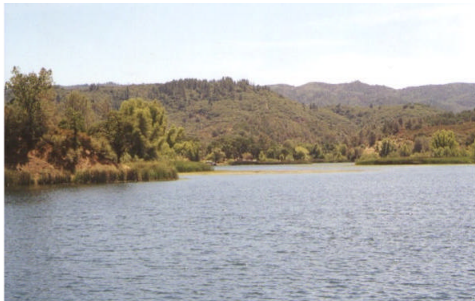
Photograph 6-2 Highland Springs Reservoir taken from the dam looking south Approx. Water Elevation El. 1461.
