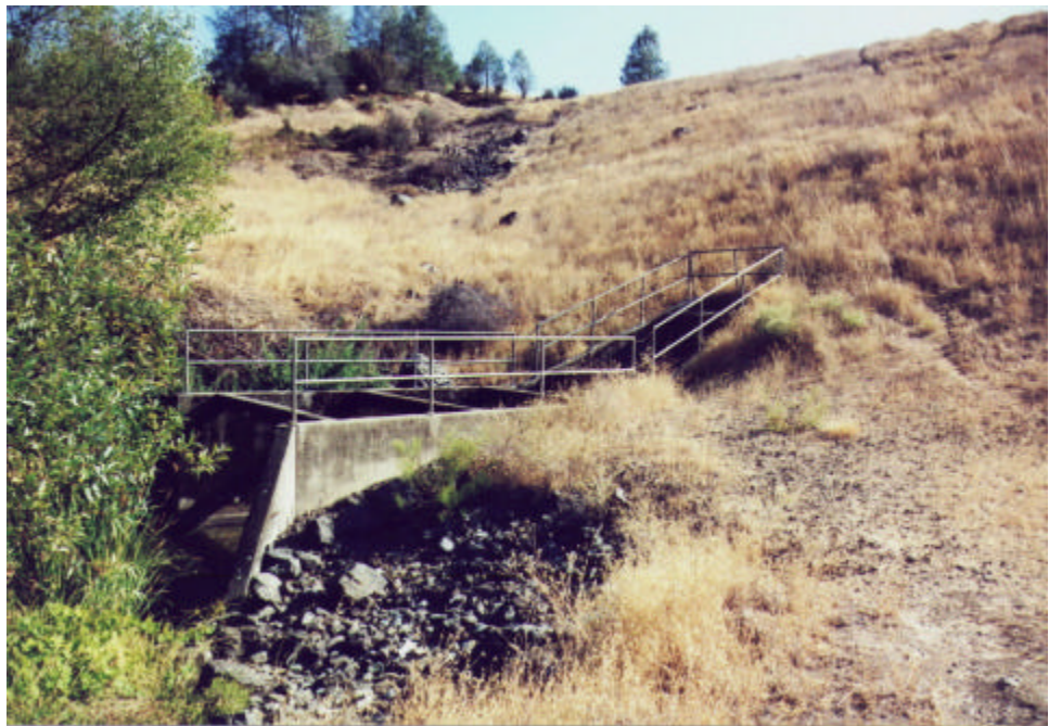
Photograph 6-7 Outlet of Principal Spillway
