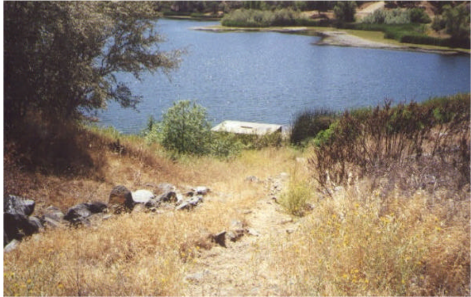
Photograph 6-6 Highland Springs Reservoir Viewed from Dam Crest showing the Principal Spillway at the east abutment
