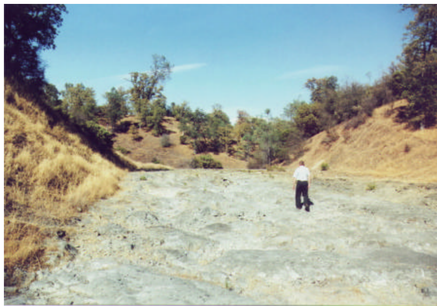
Photograph 6-8 Auxiliary Spillway Channel
