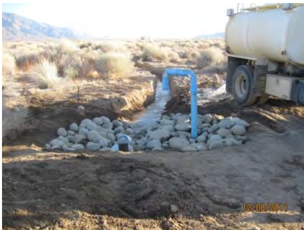
North of Mazourka Canyon Road Project, December 2011 Pipe Outfall (convergence of both pipelines) Within Exclosure During Implementation
