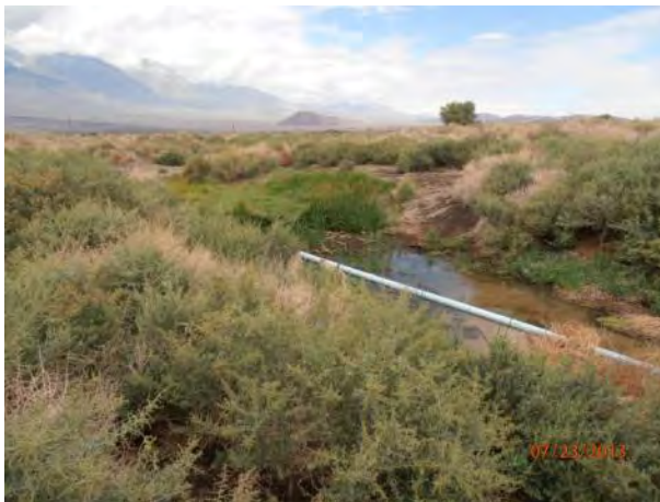
Aberdeen Ditch, July 2013 Extended Pipe Outfall
